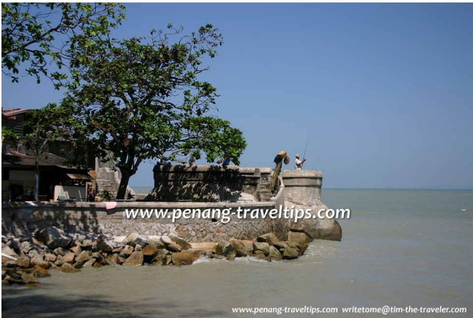
The retaining wall at Tanjong Tokong (23 December 2003)
