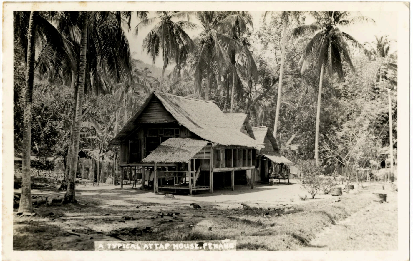
A typical attap house in Penang from the late 1950s (ML-3694). This well-structured house is separated into three parts, a front portion (with the verandah, porch and stairs), a middle portion which serves as the sleeping area, and a kitchen located at the back (as stated in A Traditional Malay House , by Abdul Halim Nasir and Wan Hashim Wan Teh).
