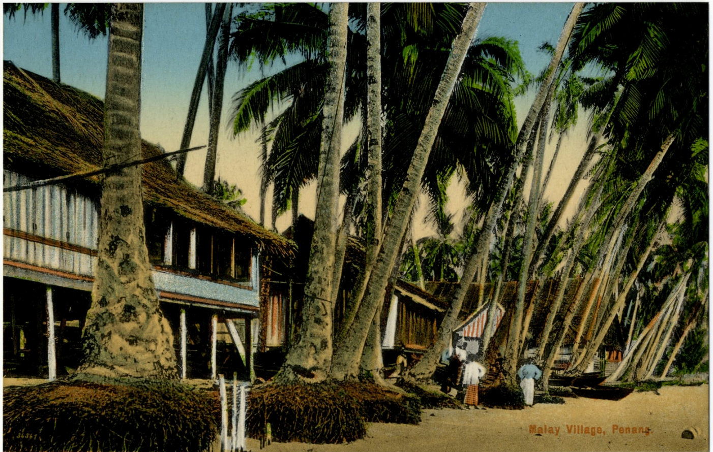
A Malay village located along North Beach, believed to be along the Bagan Jermal area c.1910 (ML-5410). Such settlements, especially those built along the coastline, consist of raised floor construction to weather the tropical climate. The space under the raised deck may be utilised for various purposes, including storage.
