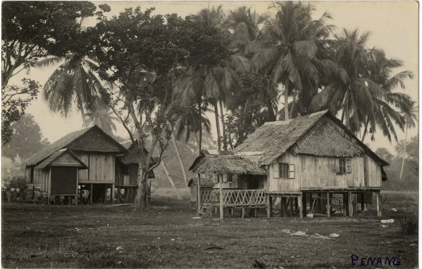
Penang Malay houses c.1920s (ML-1644). These are typical of dwellings built inland.
